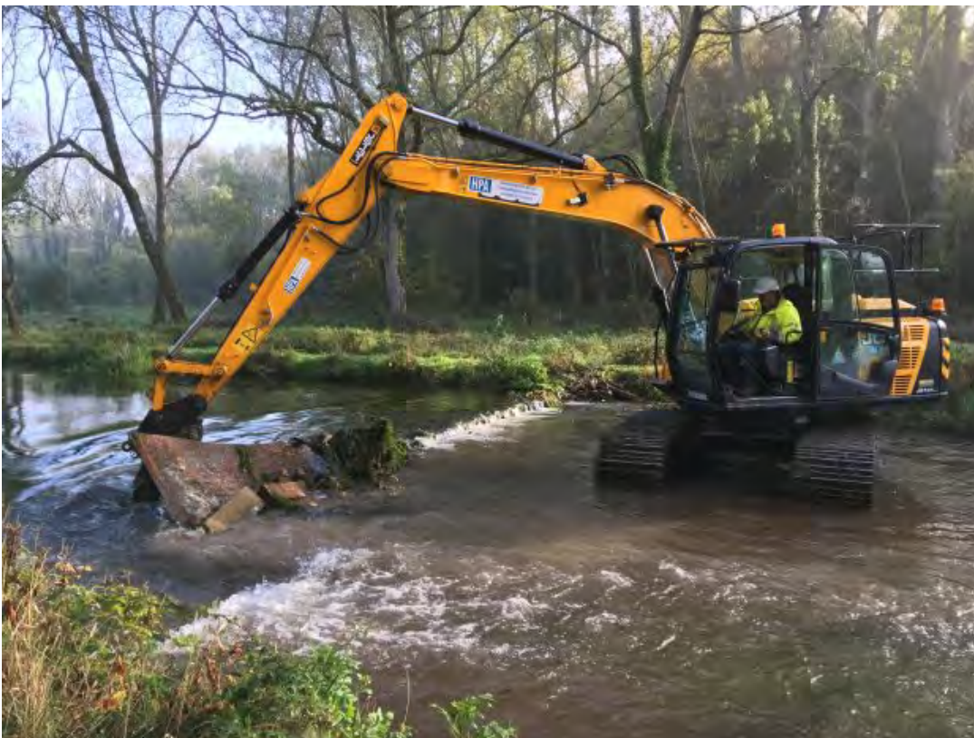
Figure 3.3: Activities as part of restoration works on the Test & Itchen
