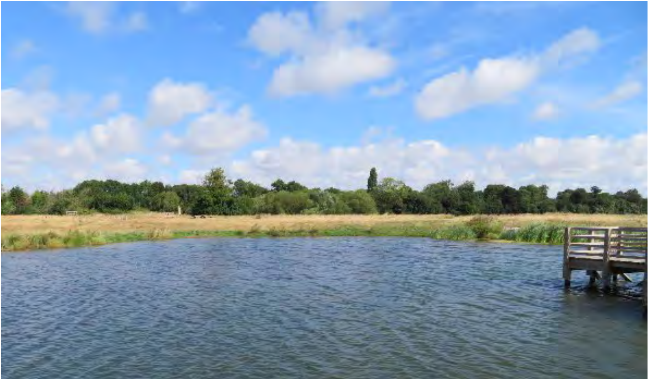
Figure 3.24: Balancing pond at Trumpington Meadows Country Park
